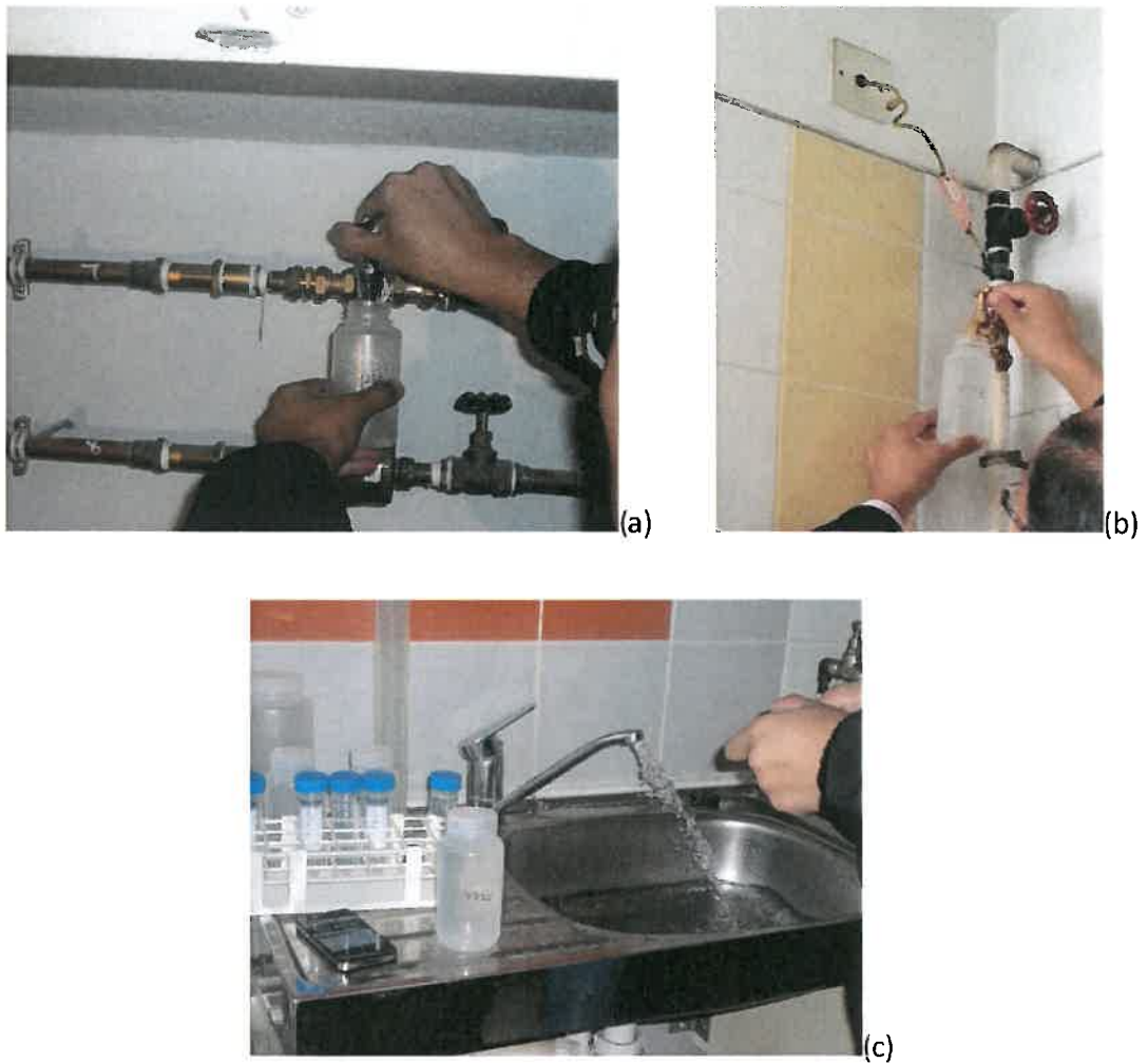
Figure V-1 Sampling at (a) installed tap in meter position; (b) tap at the water supply pipe entry to flat; and (c) kitchen tap.
